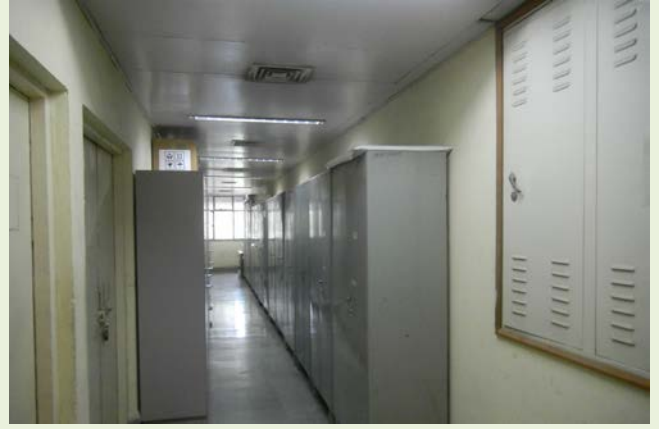
Pic 10 ACD, ADL building
